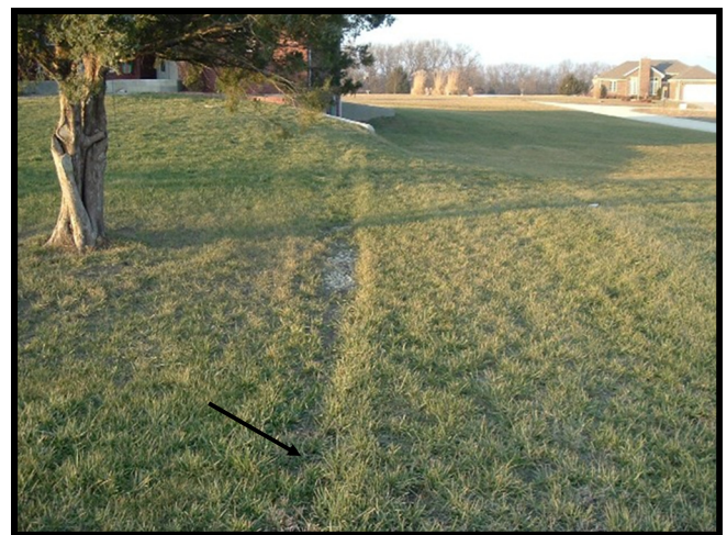
Malfunctioning curtain drain. Grass has been allowed to cover most of the gravel; water is not diverted but flows freely downhill.
