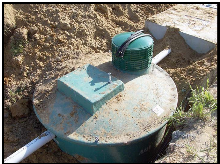
Installation of an aeration treatment unit.
