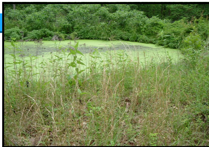
Lagoon MAINTENANCE includes cutting grass, weeds, and trees growing near the lagoon. The lagoon berm can be damaged when woody plants are allowed to grow. Duckweed growing on the water surface and grass or weeds growing over the waters edge can interfere with treatment and harbor mosquitoes.
