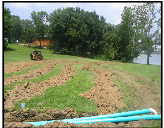
Dispersal trenches installed on contour.
