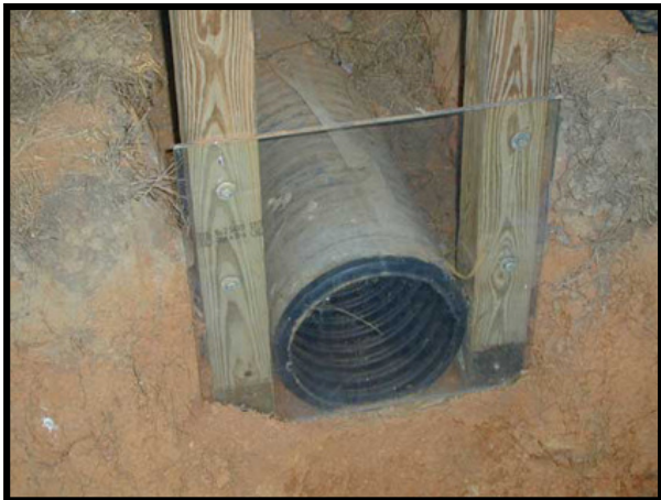
Filter wrapped 10" inch perforated corrugated pipe.
