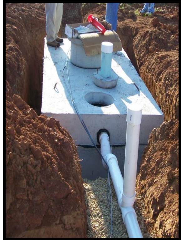
Installation of a 1,000 gallon concrete septic tank.
