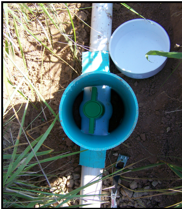
Low Pressure Pipe Valve (LPP). Valve opened to flush LPP distribution line. After flushing, valves are used to adjust the operating pressure in each LPP distribution line.
